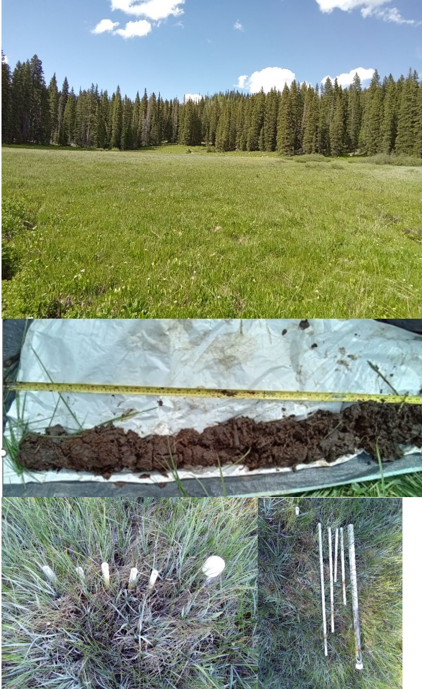
Figure 1. Grey Jay Fen (top) on the Grand Mesa (Leon Timber Sale); soil (peat) excavated to install well (center); piezometer-well nest (installed; bottom left); PVC piezometers & well prior to installation (bottom right).
